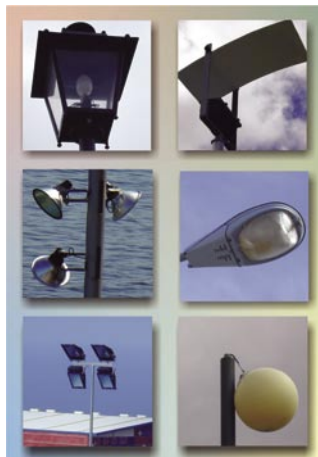
Figure 3. Lighting fixtures which do not comply with the Canary Islands Sky Law.
